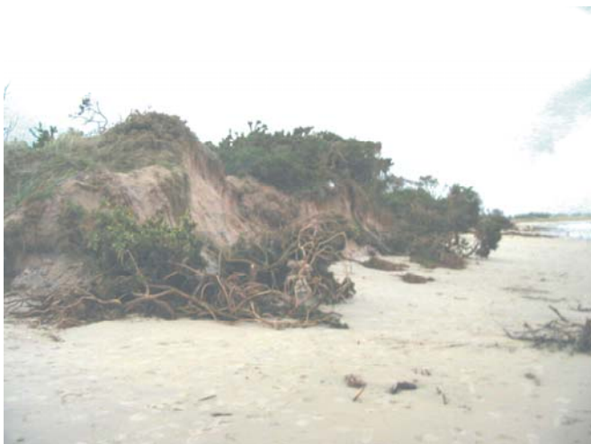
Figure 1 Storm damage at Studland, 29 October 2004
