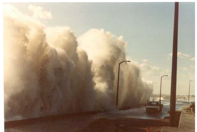
Overtopping at Sandgate 2000
