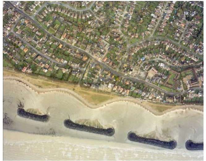
Offshore breakwaters at Elmer, West Sussex
